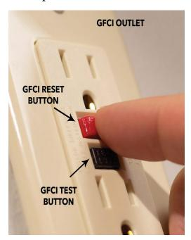
2. Upon inspection if the *Test* button is pushed all the way in, first unplug any electrical devices from the outlet. Reset the breaker by pushing the *Reset* button on the GFCE outlet.
