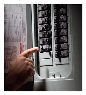
3. Should the GFCE outlet not reset upon pressing the button, go to the fuse box located within the residence and look to see if the breaker is turned off. Switch the breaker back to the *On* position, if the breaker has turned off from a surge of current.
